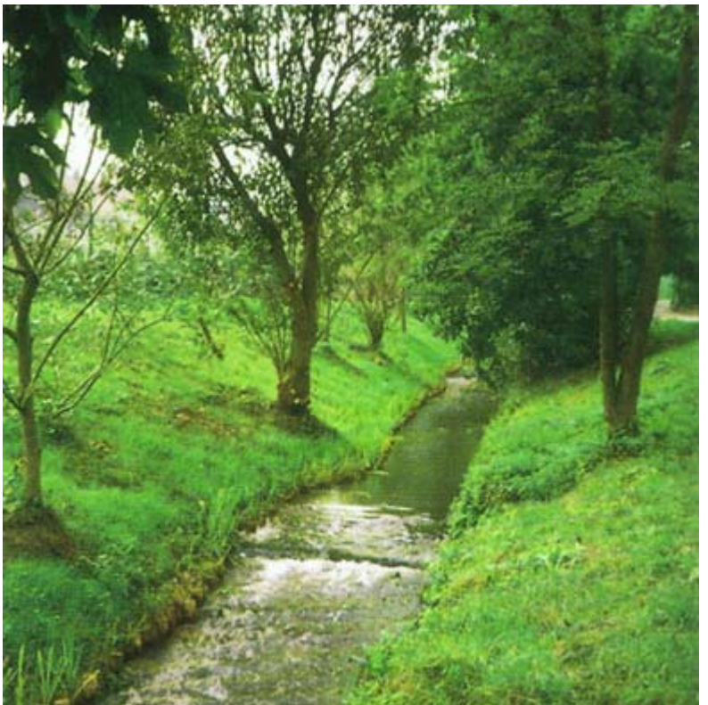
Fibre Rolls installed as a toe protection
